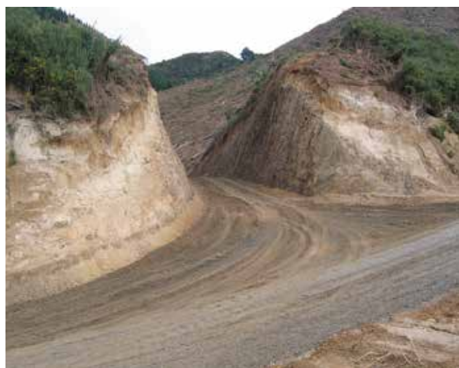
Papa/mudstone can have steep batter slopes which also reduce the volume of material that needs to be moved
