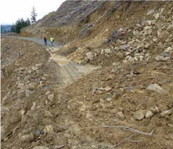
Left: Ditches initially need regular maintenance, especially where cut bank collapse is a common and unwanted aspect in some soil and geology types. Right: Poor ditch maintenance caused a scour across this road
