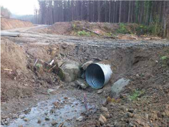
Example of a corrugated pipe culvert across a small waterway
