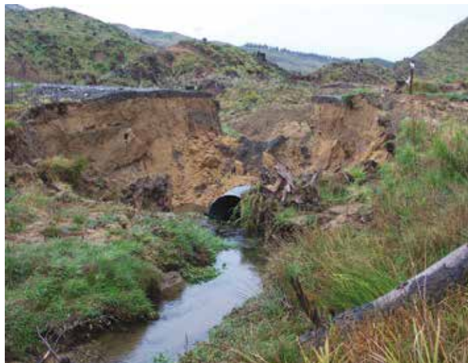
Left: A well-functioning spillway that protected the road when logging debris, mobilised by a 1-in-50-year storm, blocked the culvert mouth. Right: An expensive, inconvenient problem with potential environmental and downstream impacts. This pipe culvert failed when it was blocked by woody debris
