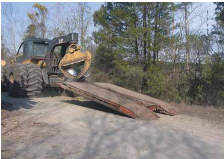
A temporary steel crossing
