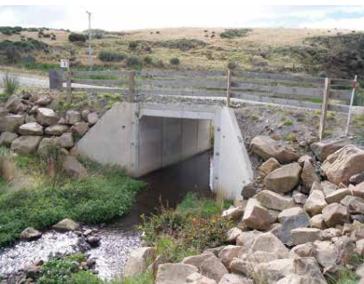
Example of a large concrete box culvert
