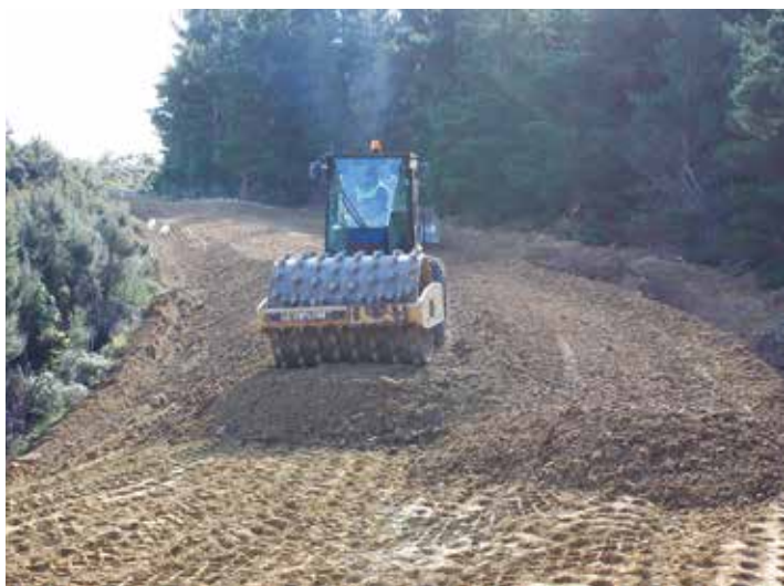
Compaction needs to be done in layers
