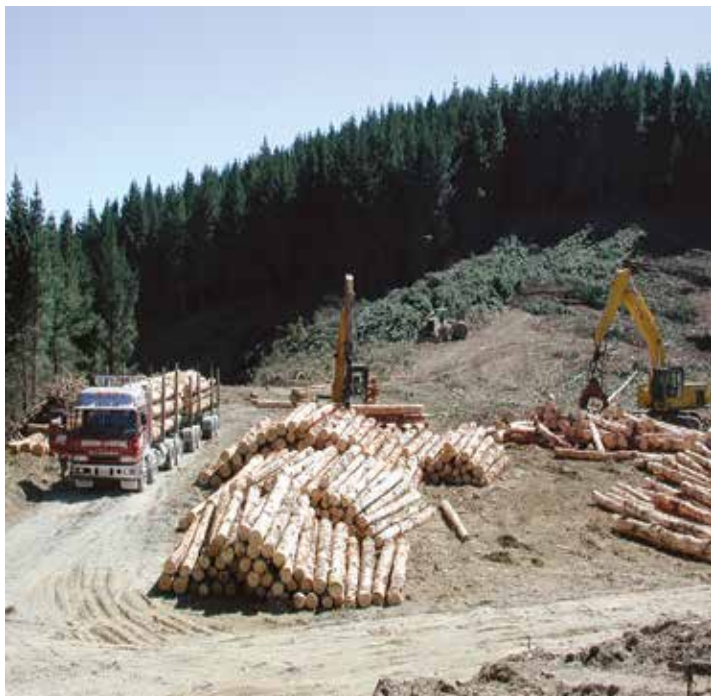
Roadside landings provide a clear separation between landing activities and the road, but can require more effort to reach logs stacks when loading out
