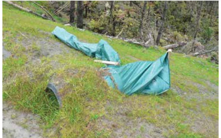
Left: Culvert sock securely attached to culvert and anchored. Right: A poorly designed and secured sock; the inlet has been bypassed and the wind has twisted it
