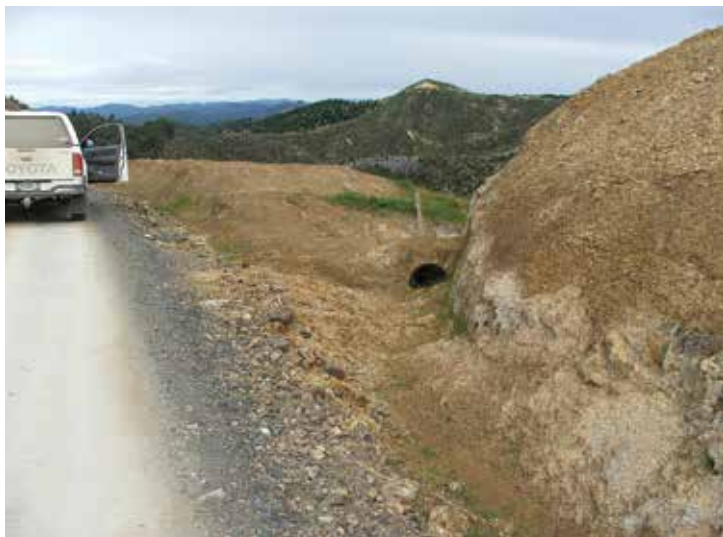
Left: Cut-out leading to a flume. Right: Cut-outs with water bars and now-filled sediment traps on a decommissioned road
