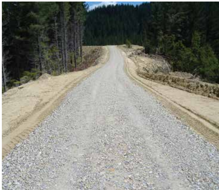
A typical one-lane secondary road. The widened shoulder on the left provides room to allow opposing traffic to pass
