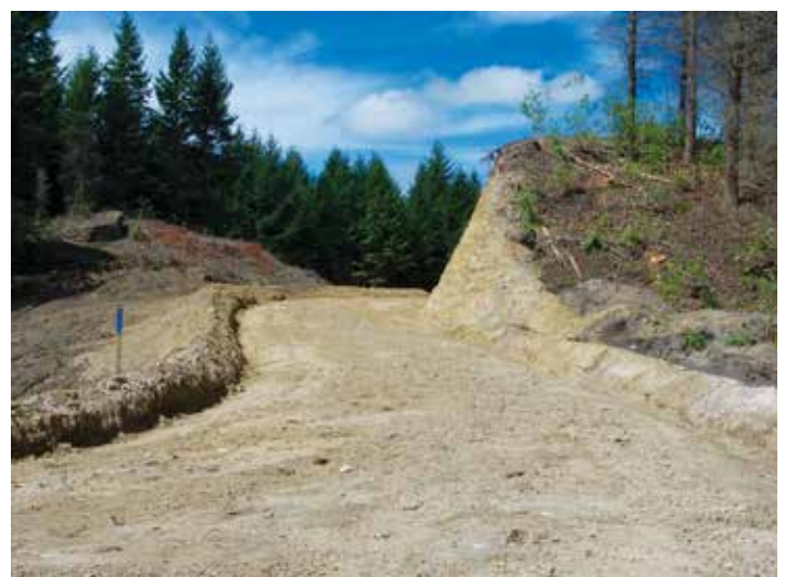
Well-prepared, compacted and shaped subgrade ready for placement of aggregate
