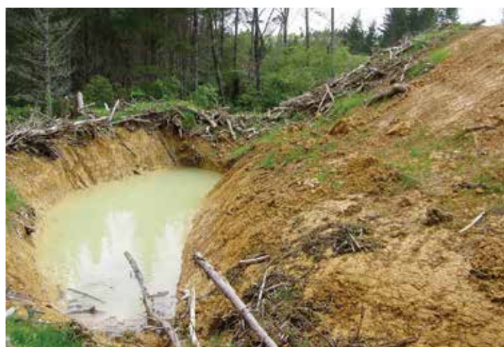
Left: A poorly constructed sediment pond. It is located on fill, is not level, and both the inlet and outlet are scoured. The lowest part of the pond is almost at outlet level. This could completely fail if water overtopped it. Right: A well-constructed pond draining a landing. It is constructed in the hard. It may become challenging to protect the structure during the harvesting phase as it is incorporated within the landing. Both structures require maintenance, so should be accessible
