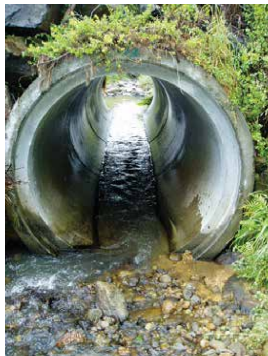
Examples of smooth-bore concrete pipe culverts with and without wingwalls. The photo below demonstrates the potential issue of fish passage, due to high water velocity
