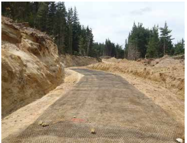
Geogrid laid on a subgrade prior to application of the aggregate layer
