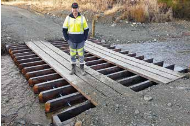
A portable temporary bridge specifically designed to accommodate truck traffic. This will be a cost-effective crossing when used in the right location
