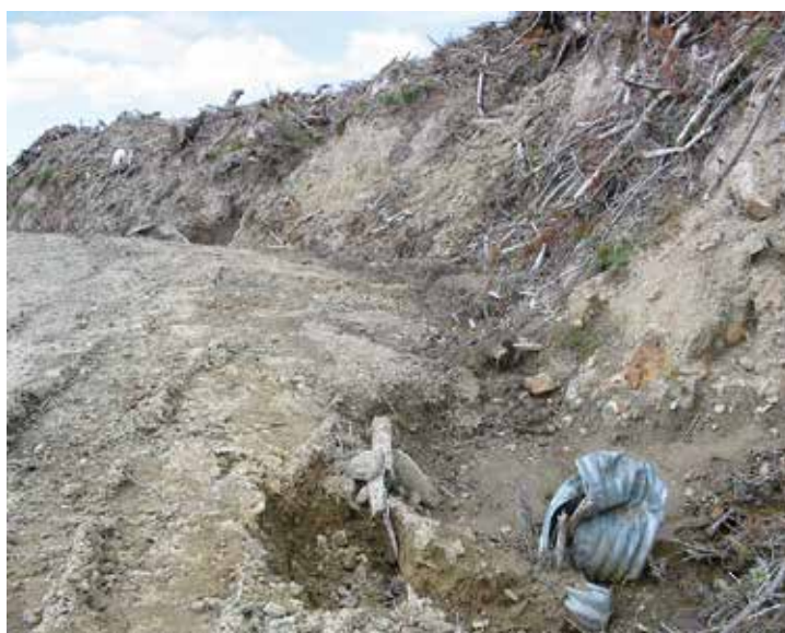
Check for crushed drainage culverts after logging. Drainage culverts are easily damaged if the maintenance operator is inattentive
