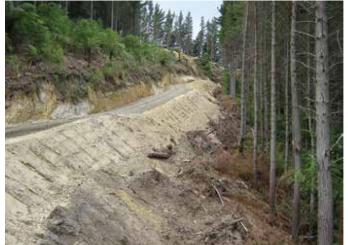
Well-constructed road with good salvage width and construction techniques
