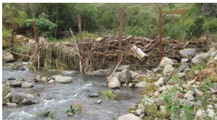
This highly effective debris trap needs to be cleaned to continue to limit slash from going off-site. Know the NES-PF regulations around debris trap maintenance and reporting
