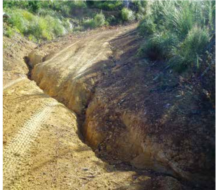
Left: Ditches initially need regular maintenance, especially where cut bank collapse is a common and unwanted aspect in some soil and geology types. Right: Poor ditch maintenance caused a scour across this road
