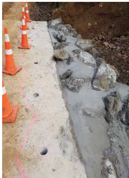
This battery culvert was well constructed, and had relatively minor repairs and maintenance considering the storm flow was 1.5 m above the structure. Left: The reno mattress has protected the crossing from undermining. Note that the gravel movement from the storm has blocked all but one of the pipes. Right: Weaknesses have been armoured. The holes are used to pump grout in and fill the void. Armour known weaknesses
