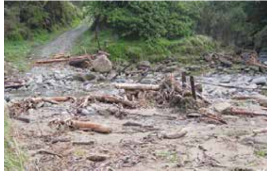
Left: Radiata stumps are not preferred anchors, as many will have lost their tensile strength within the design life of the structure. Right: There was too much energy in the river and the structure failed. The storm flow moved large boulders, as can be seen of the far river bank. Consider putting traps in side creeks or where the river's energy lowers
