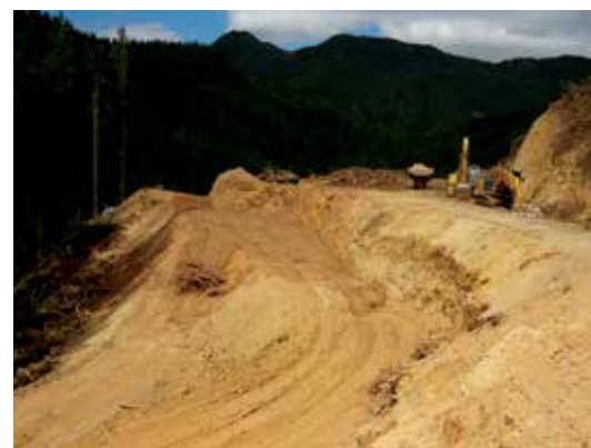
Above: Balancing cuts and fills help minimise the overall earthworks required to construct a forest road Below: Landings can generate large volumes of earthworks. Benching is essential in anything other than the easiest country to help stabilise the fill
