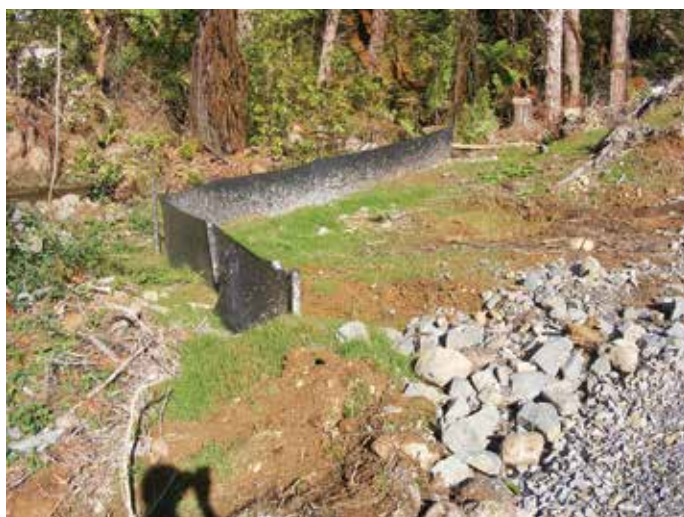
Two well-constructed applications for sediment fences
