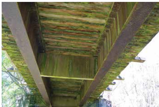
Regularly inspect the condition of bridge components
