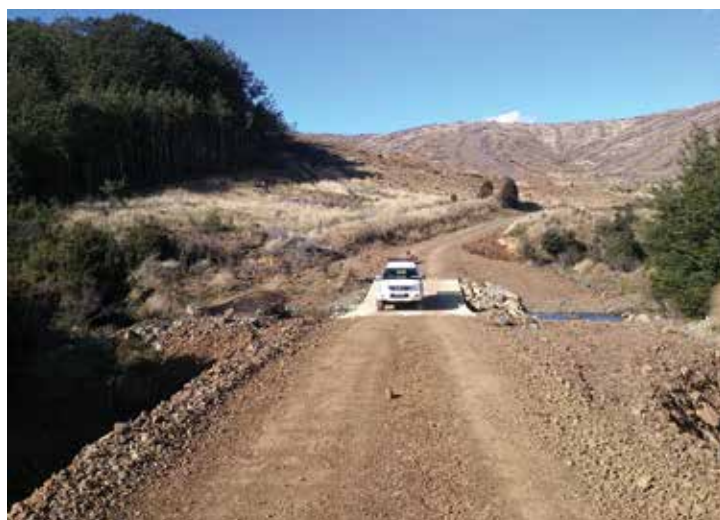
Left: A well-constructed drift deck. Right: A drift deck crossing, with a secondary crossing for tracked logging machines that would damage the concrete pad
