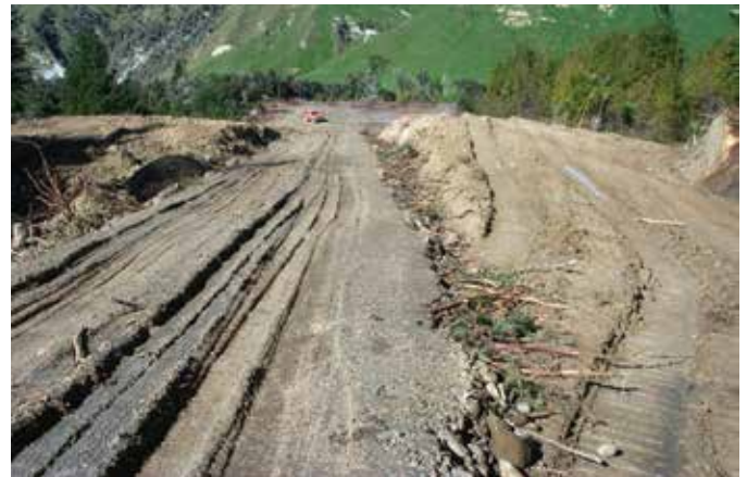
Slash corduroy provided truck access on a step section of road after the subgrade failed
