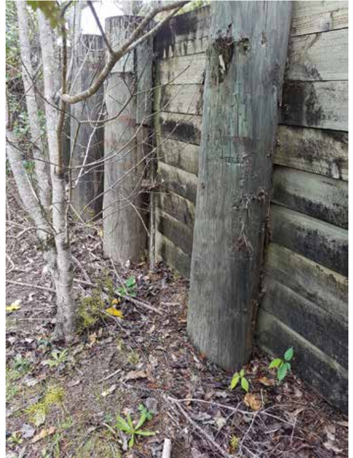
Timber cantilever retaining wall
