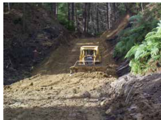
Above: Balancing cuts and fills help minimise the overall earthworks required to construct a forest road Below: Landings can generate large volumes of earthworks. Benching is essential in anything other than the easiest country to help stabilise the fill
