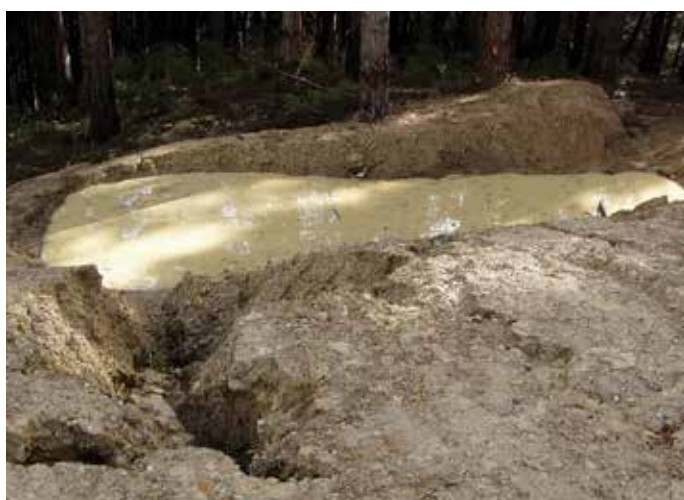
Left: A poorly constructed sediment pond. It is located on fill, is not level, and both the inlet and outlet are scoured. The lowest part of the pond is almost at outlet level. This could completely fail if water overtopped it. Right: A well-constructed pond draining a landing. It is constructed in the hard. It may become challenging to protect the structure during the harvesting phase as it is incorporated within the landing. Both structures require maintenance, so should be accessible
