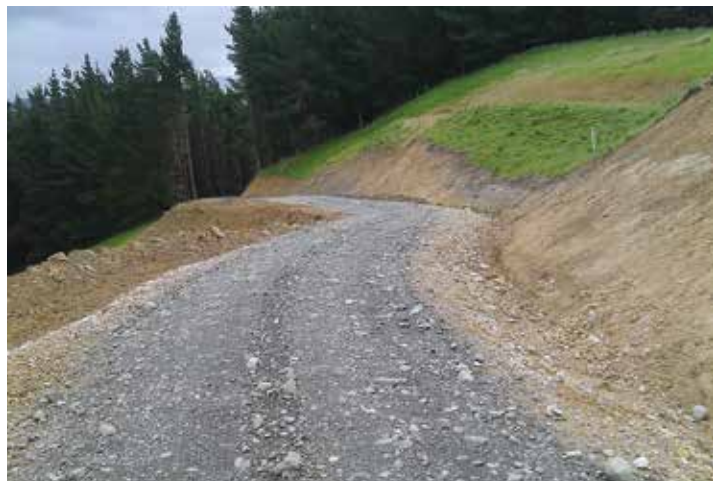
Cut and side cast construction
