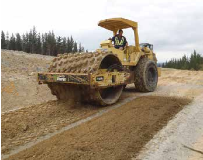
Sheep-foot roller preparing the subgrade of a new forest road
