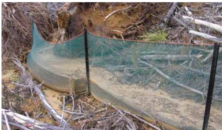
Well-functioning fences. They have captured most of the larger sediment and have not failed, despite containing a significant weight of material. Right: Maintenance is required for the shade cloth fence
