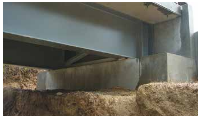
Steel truss, concrete slab bridge
