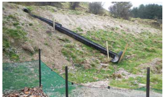
An effective way to reduce sediment is to use an energy dissipater like slash, rock or a short section of flume perpendicular at the exit, in conjunction with a silt fence
