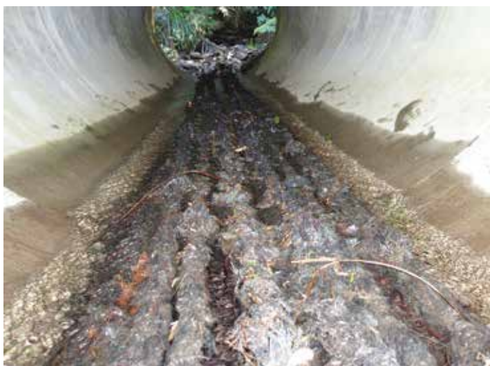
Mussel spat ropes are the most cost-effective solution for fish passage. (Credit: Bruno David, Waikato Regional Council)
