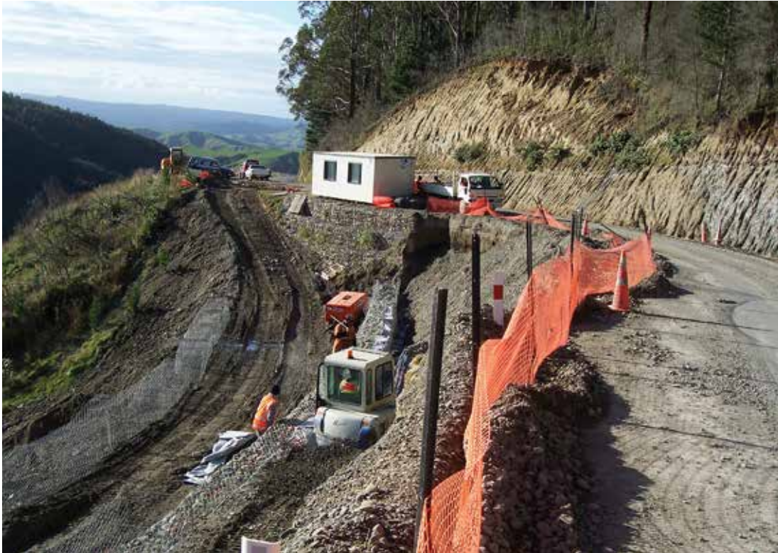
Gabion wall being constructed to support a fill slope
