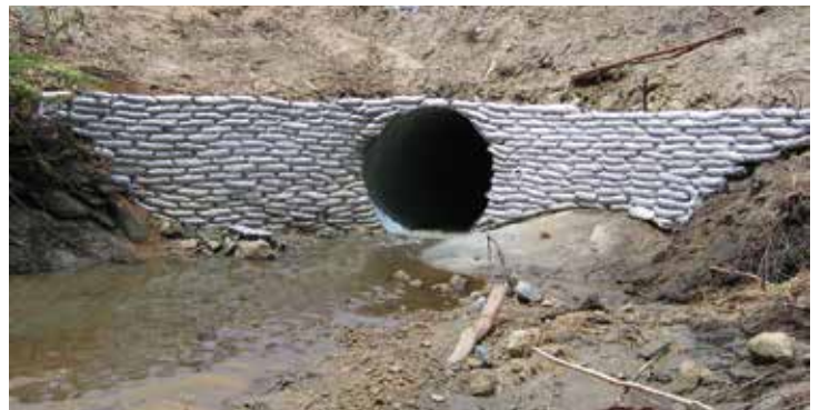
The large culvert with bagged cement and sandbag headwall has been designed to resist scour in debris laden flood flows
