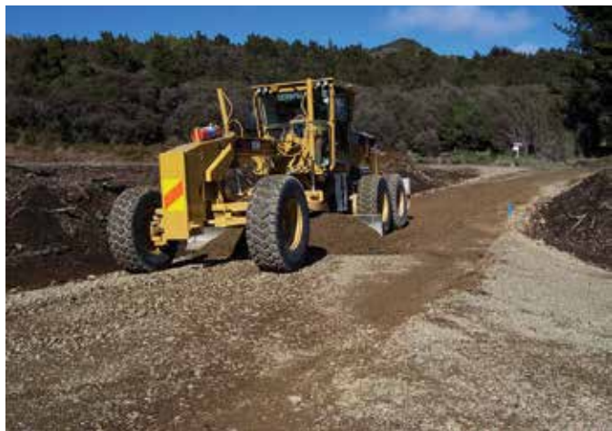
Grader reshaping road pavement
