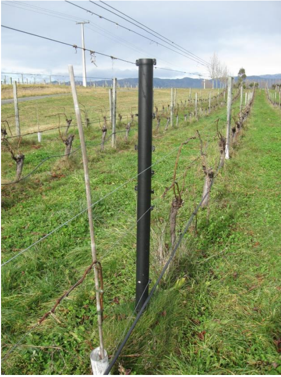
Figure 25: WoodSheild post manufactured by Fosters in vineyard 4a. This is an untreated pine peeler core encased in 6mm thick of black polyethylene to produce a finished size of 83mm trellis post.
