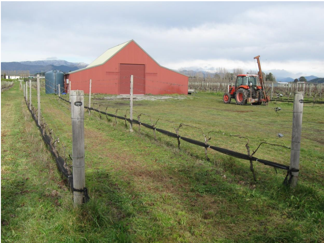
Figure 27: View at vineyard 4a of small vineyard area with E. globoidea trellis posts and Wallaba strainers. Wallaba are imported naturally durable posts that were available in Marlborough through local rural supply agents. This small area of vineyard was part of the in ground post assessment.
