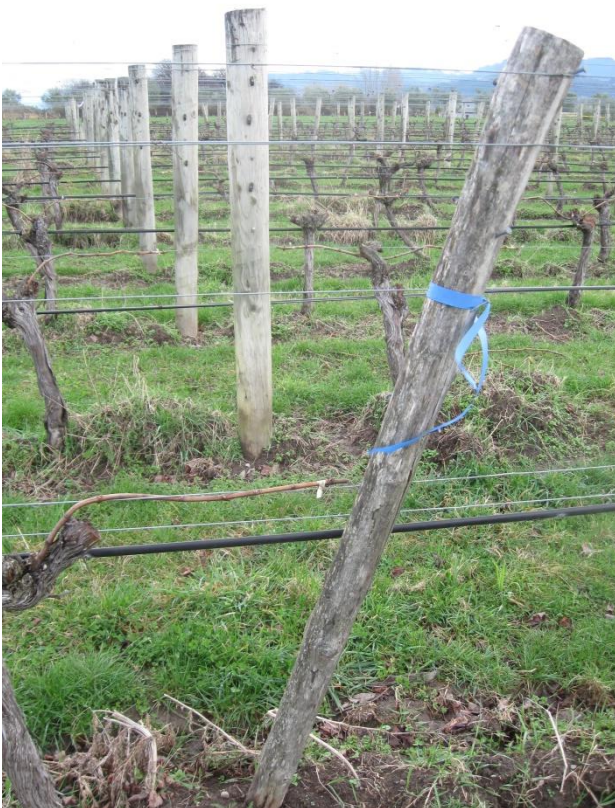
Figure 30: Imported teak round post decayed at just below ground level and marked for replacement in vineyard 5.
