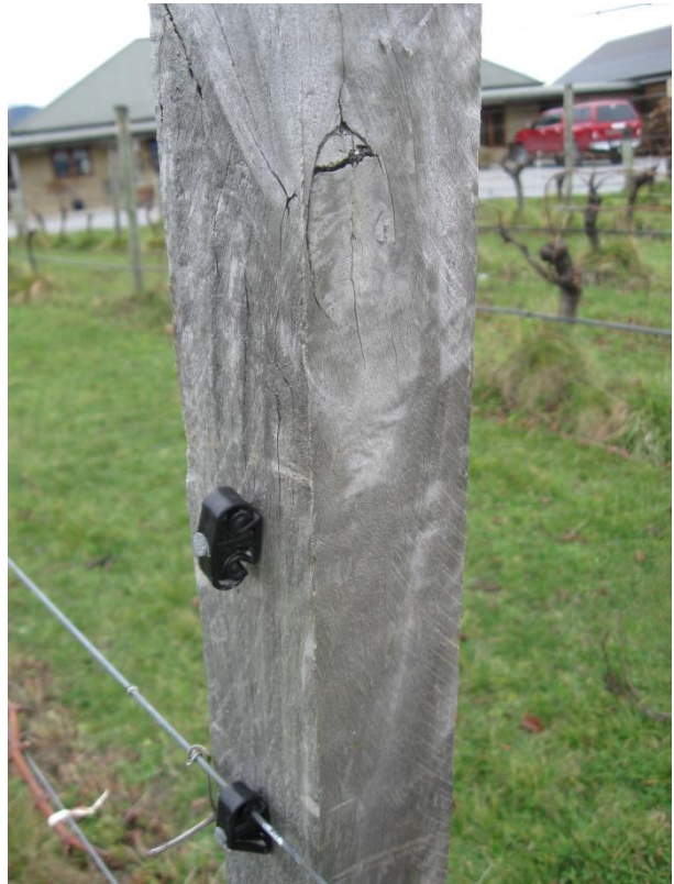
Figure 24: E. globoidea showing wire hangers fastened with clouts at vineyard 4c. Note the size of the spike knot.
