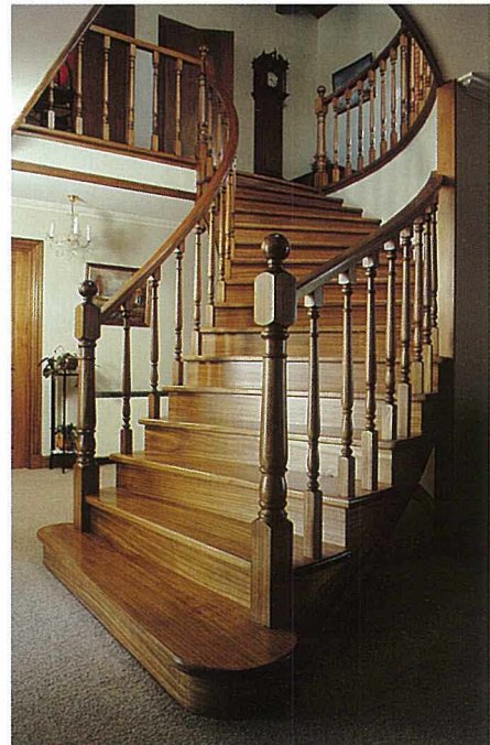
FIG. 28 —Staircase and joinery made from E. fastigata .
