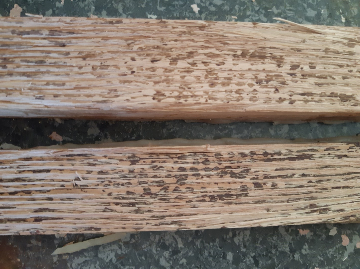
Figure 10. Poor glue spread on veneers
