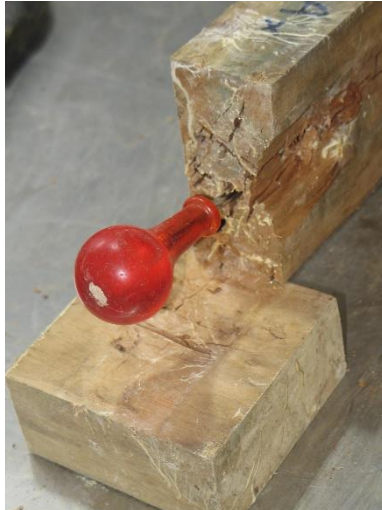
Figure 7: Severe decay in the joint of a heartwood/sapwood Eucalyptus regnans sample after twenty-four months exposure (sample 418).
