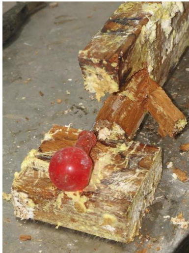
Figure 5: Severe decay in the joint of a Douglas fir heartwood sample after twenty-four months exposure (sample 502).
