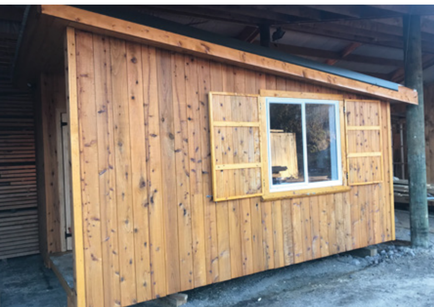
Above left: Cryptomeria japonica at the Holt arboretum, Hawke's Bay. Above right: Cryptomeria japonica timber. Below: Cabin with C. japonica shiplap cladding.
