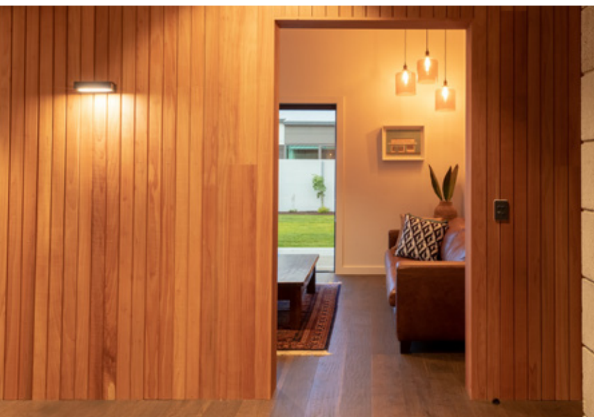
Above right and below: Sequoia sempervirens interior panelling and sarking in a Hawke's Bay house.
